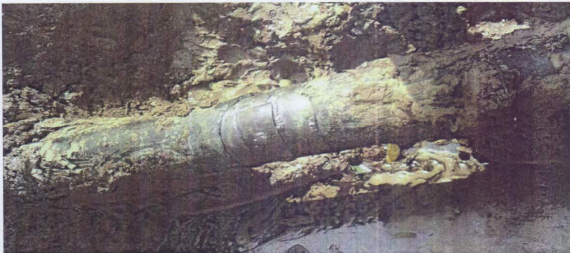
Figure 2.3. Incident point before excavation.
